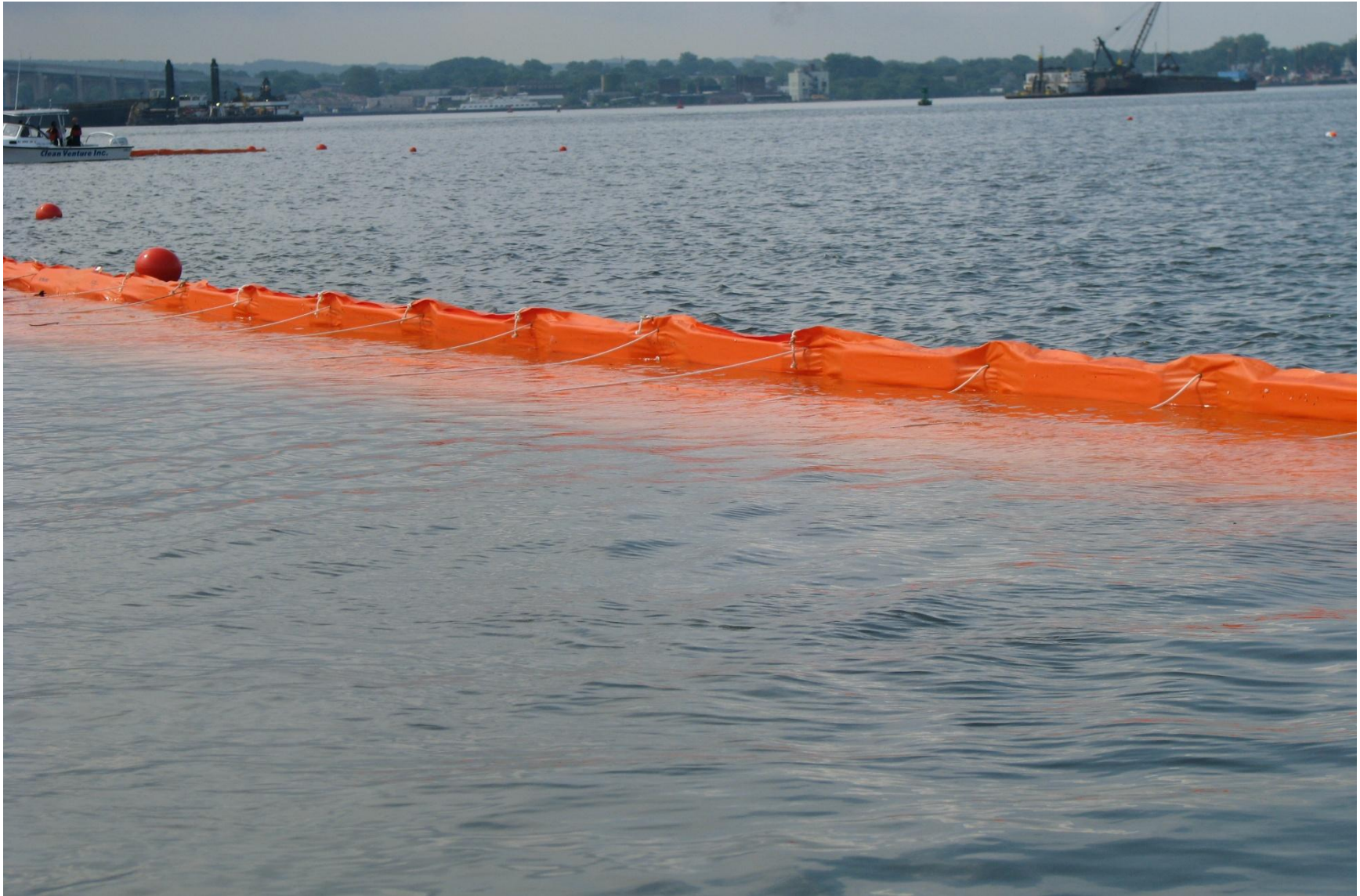
Figure 3-2. Unfurling of the silt curtain. Tidal forces are beginning to push the curtain to the surface.
