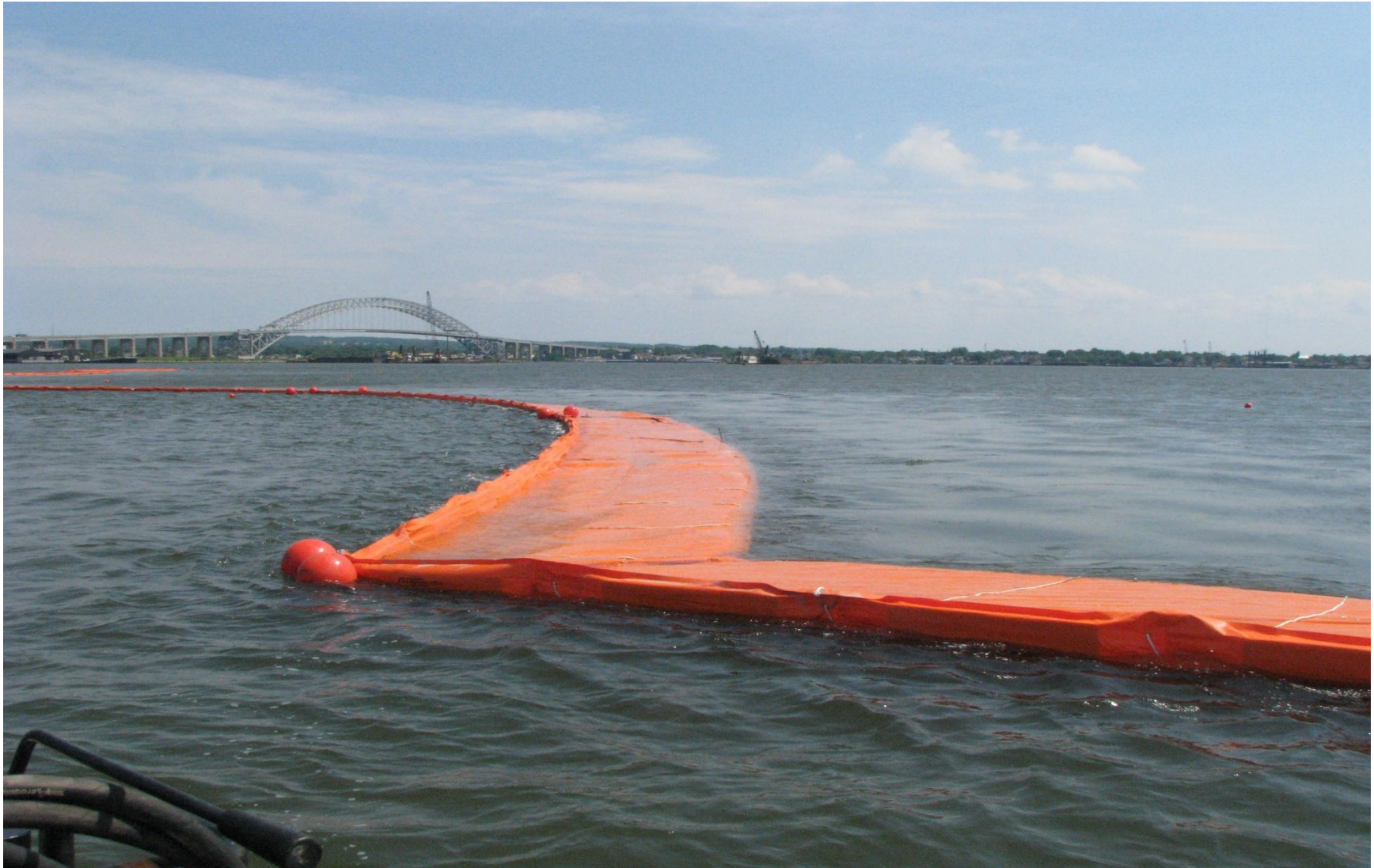
Figure 3-3. An example of silt curtain “flaring” due to current.
