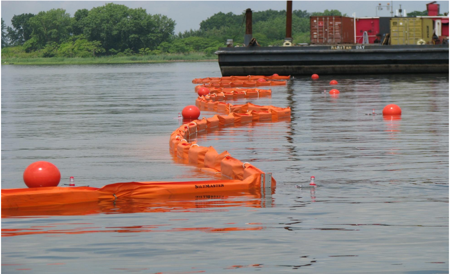
Figure 3-4. The inner most section of the silt curtain deployed at the NW end of the SEC where current velocities are lowest. Although initially deployed in a straight line, the curtain is deformed by current flow.
