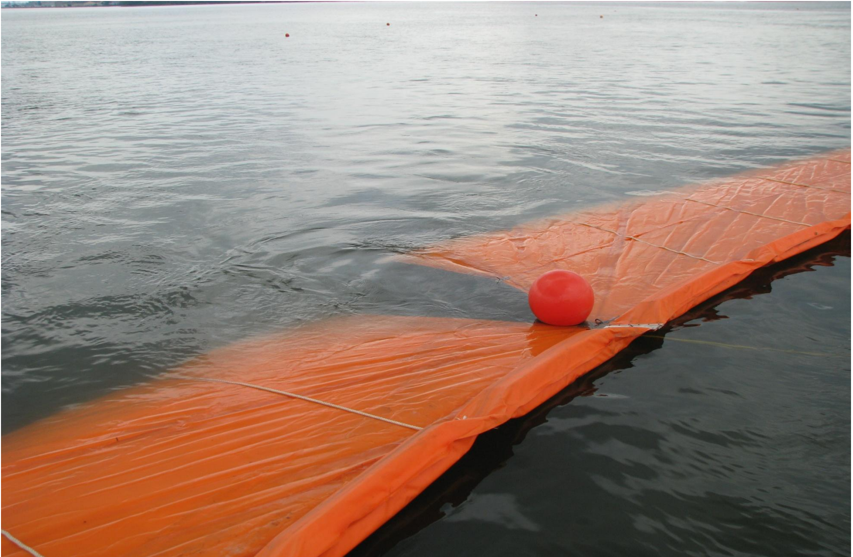
Figure 4-1. Silt curtain separating and flaring by tidal forces.
