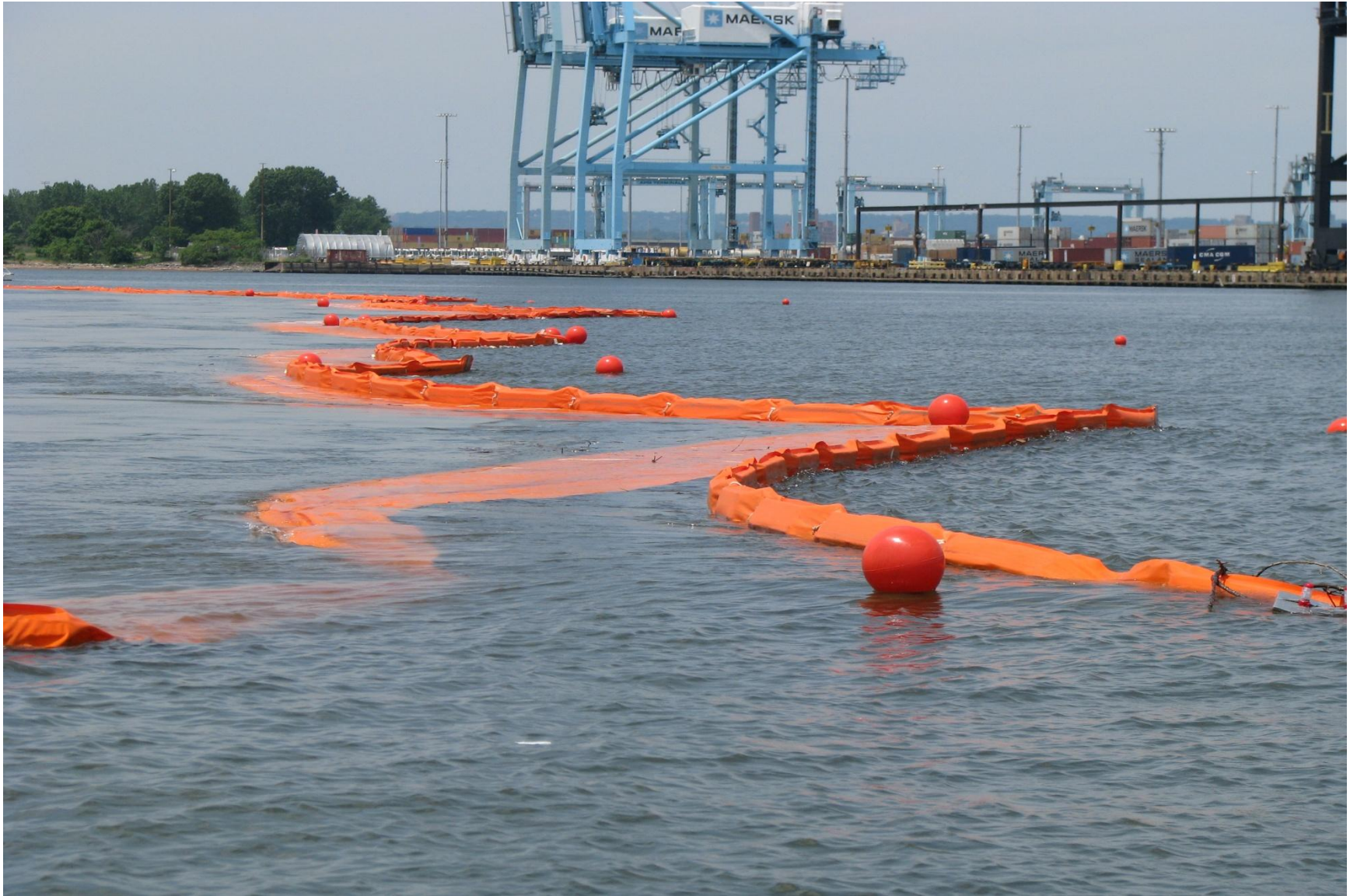
Figure 3-7. A section of the silt curtain damaged and pulled away from the boom.
