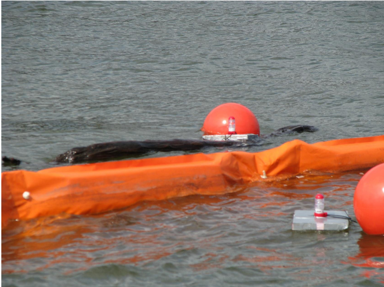
Figure E-3. Large debris, such as logs, caused structural damage to the curtain.
