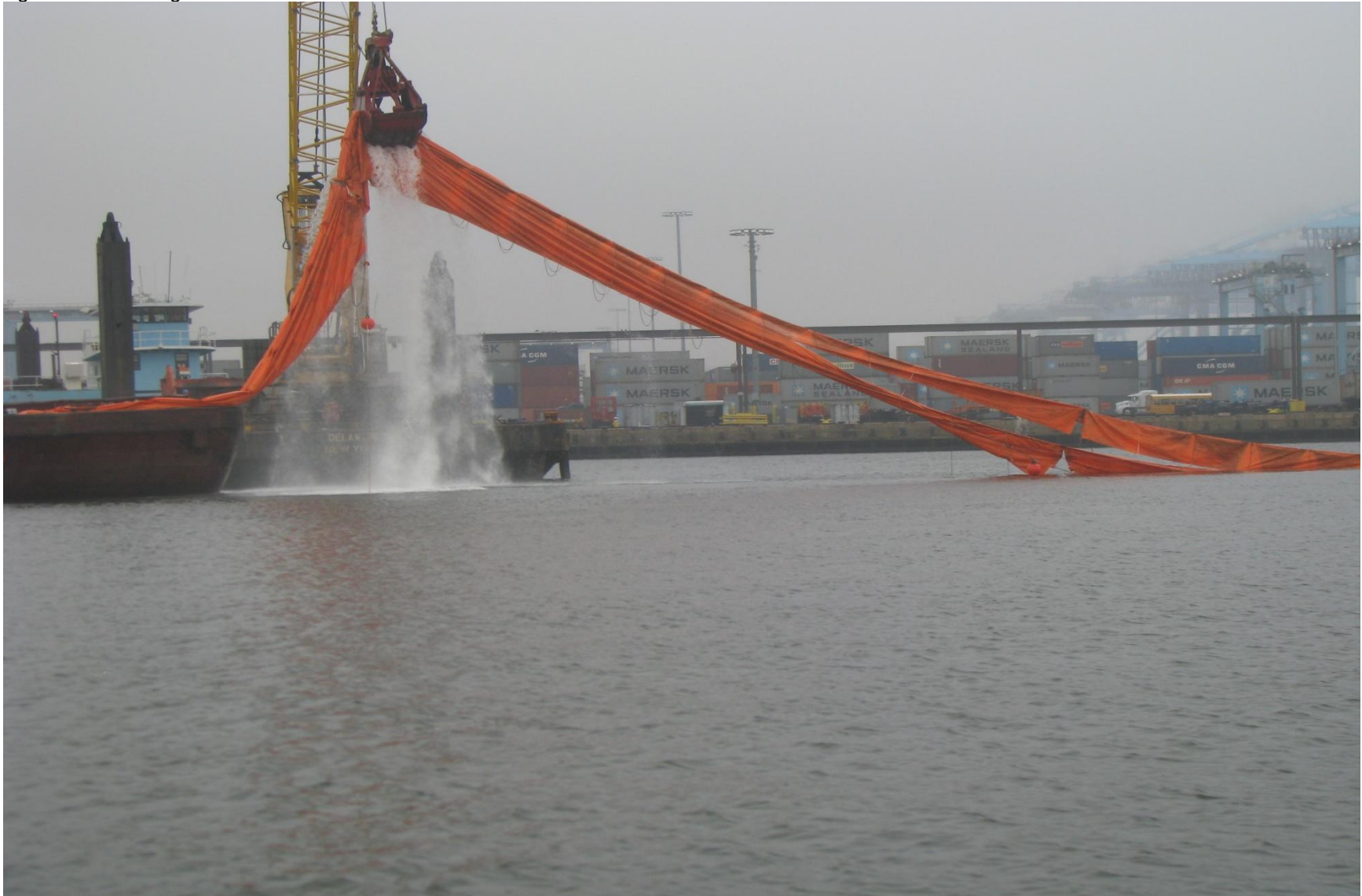
Figure 3-6. A section of the damaged silt curtain is shown during silt curtain removal.
